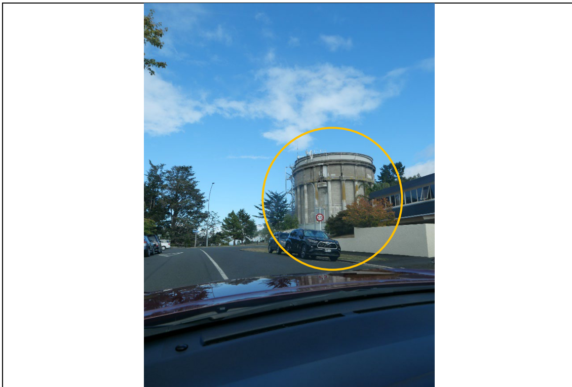
View E: a view towards the water tower from Clarence Street (heading south) The water tower is circled.
