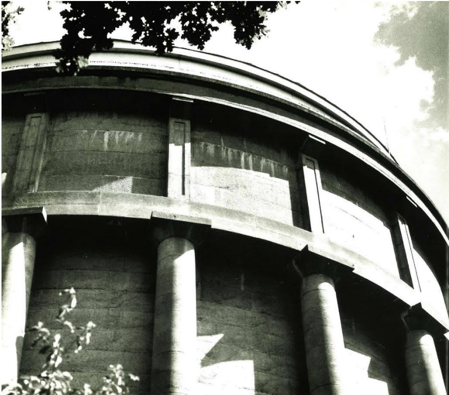
Figure 1: Water Tower, Ruakiwi Road, Hamilton. Image credits: Thornton, Geoffrey Cast in Concrete , 1996, p218, Reed Books, Auckland
