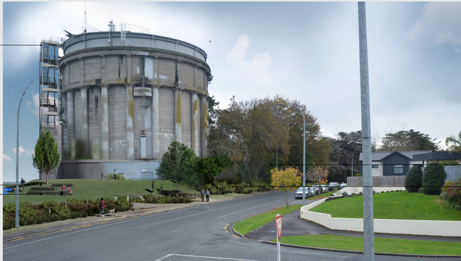
comms services and stairs retained
