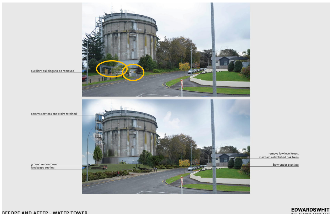
Figure 4: Non-original and non-heritage ancillary elements that could be removed (circled) to enhance the values of the heritage reservoir in hand with the proposed landscaping. Image: Edwards White Architects
